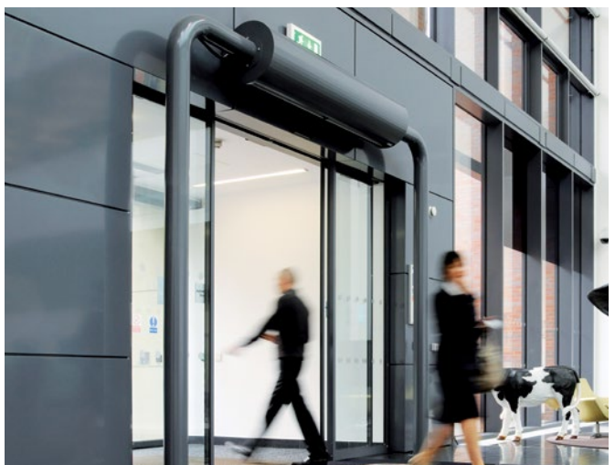
Rund Installation with special goalpost supports
