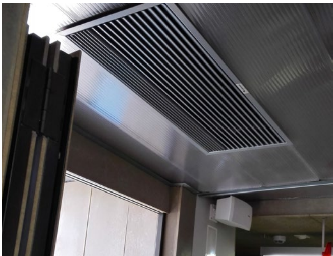
Recessed Optima Designed to install in false ceiling, custom finishes
