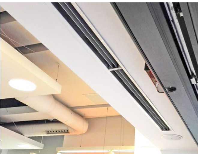
Invisair Fully invisible horizontal installation integrated in a bulkhead
