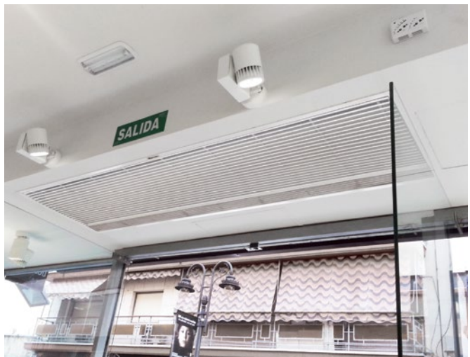
Recessed Dam Model with exposed inlet grille
