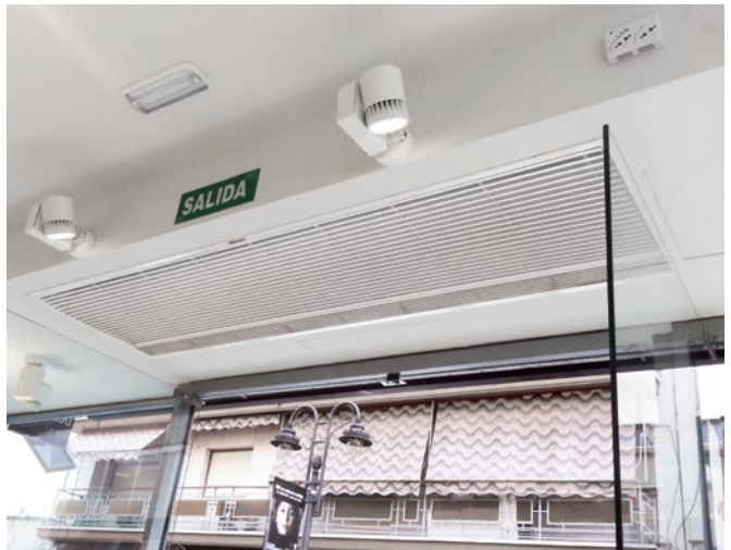
Recessed Dam Model with exposed inlet grille
