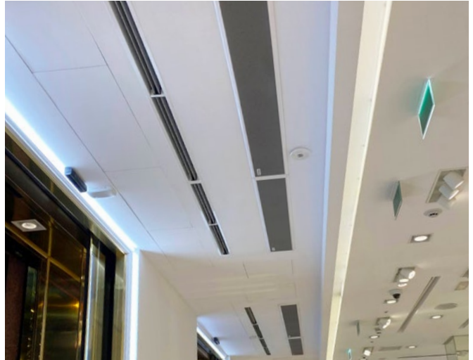
Windbox M,G Invisible installation with false ceiling kit
